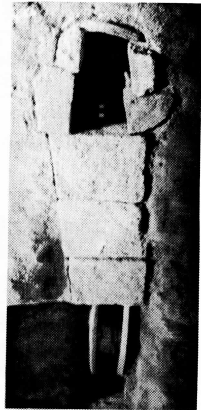
Fig. 38 Sewer installation in Building B
